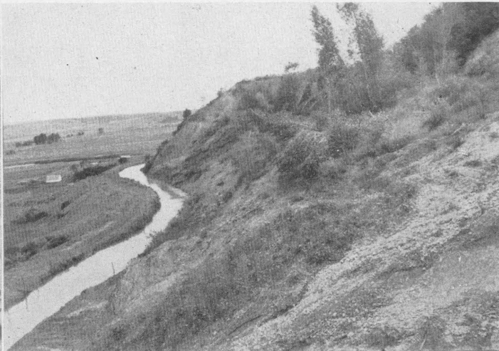
Washing and sliding of this side hill into the canal because of excessive seepage from above, and the high water table has cost the irrigators large sums for repairs and also endangered their crops (Photo by C. W. Lauritzen)
